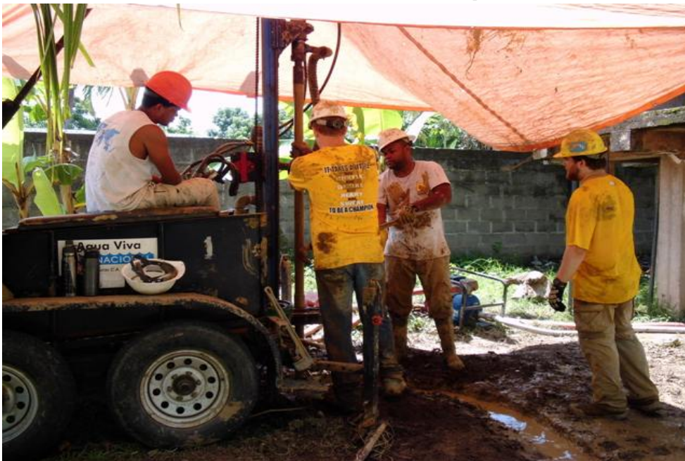
The Living Water Honduras team drilling the new borehole for the community.
