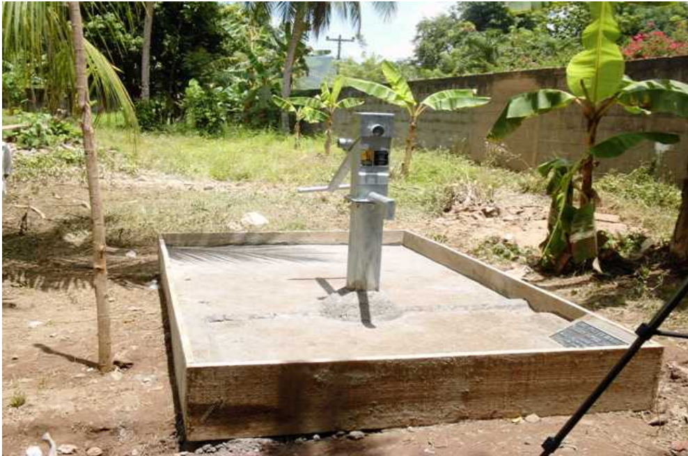
The completed water project with cement base, Afridev hand pump, and plaque.
