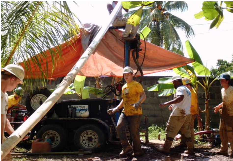
The Living Water Honduras drilling team get ready to install the PVC pipe into the well.
