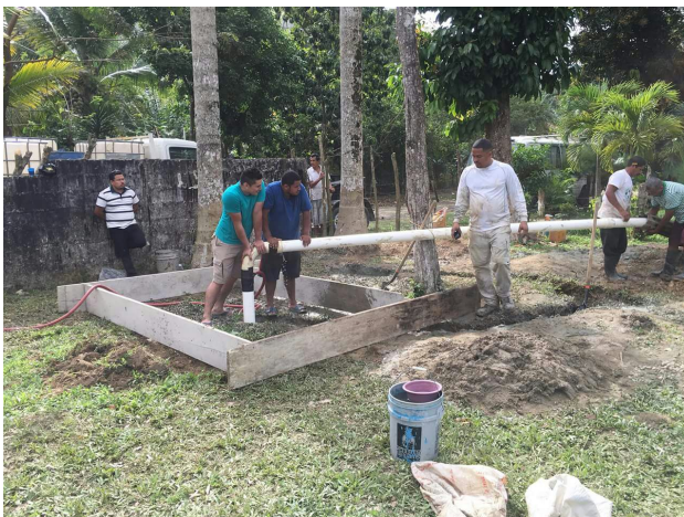
The Living Water staff case the borehole with PVC.
