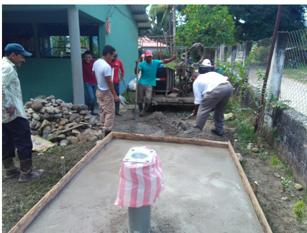
Once the borehole is cased, the team works on installing the well head.
